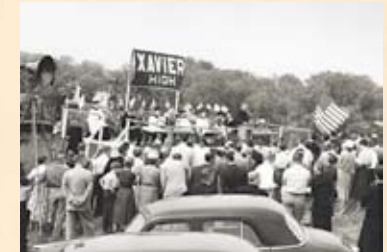
1958 groundbreaking, St. Xavier High School’s new campus in Cincinnati.
